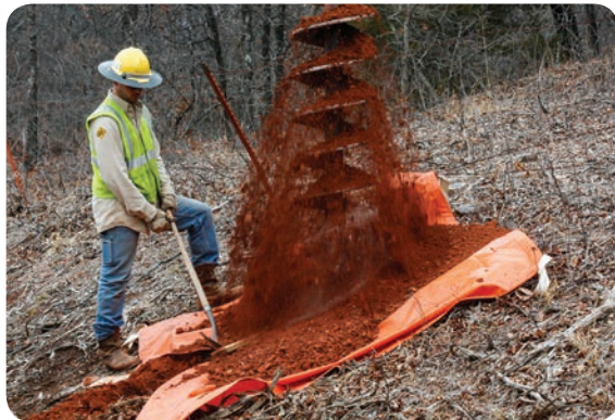
RDB-8x8-22V in Action Installing a Utility Pole
