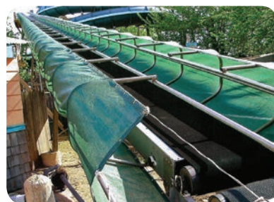
Machinery Protective Barrier (Water Park Conveyor Belt)
